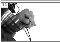
Make wire connections to power source using wire nuts provided. Make sure that no filiments are outside of the wirenut. After making the wire connections, the wires should be spread apart with the grounded conductor and the equipment-grounding conductor on one side of the outlet box and ungrounded conductor on the other side of the outlet box.
